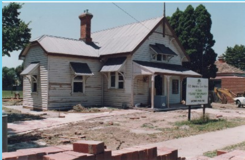
Restoration work on the Court House in 1993 by Peter Free
